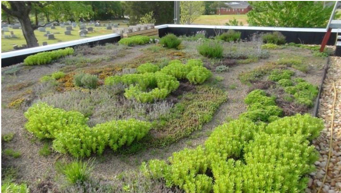
Figure 4.36 View facing southeast on OCHM green roof, April 2014
