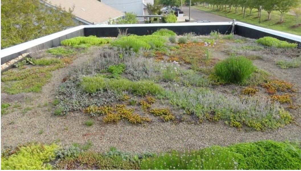
Figure 4.35 View facing north on OCHM green roof, April 2014
