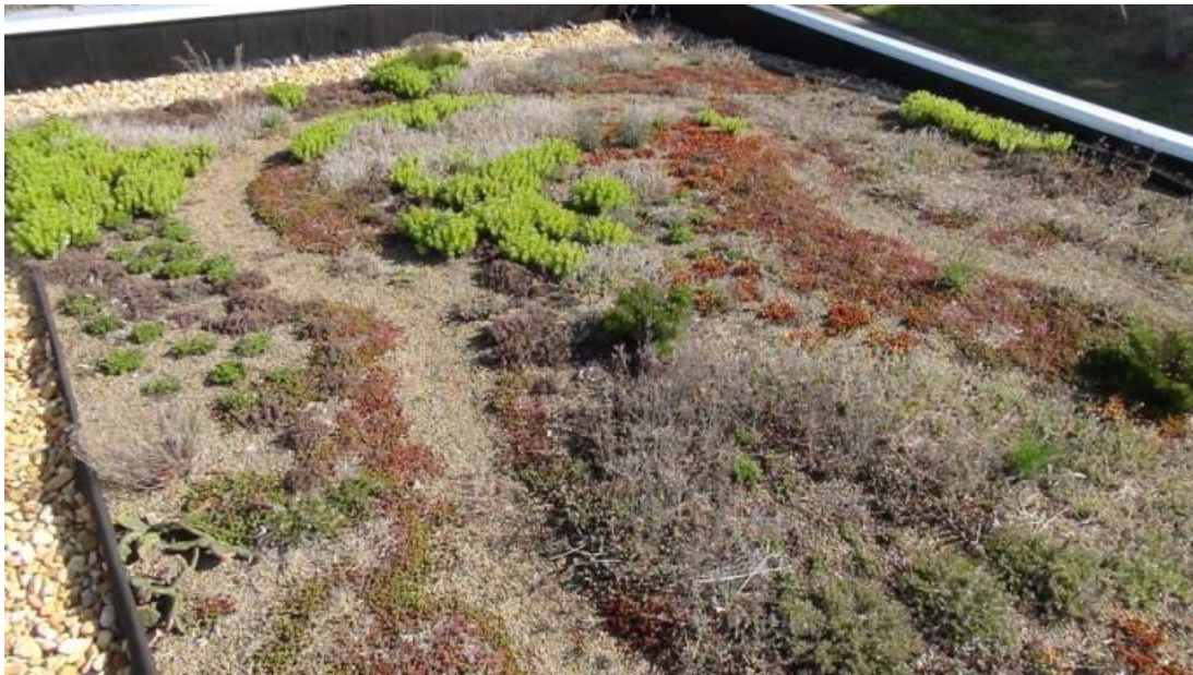
Figure 4.32 View facing northeast on OCHM green roof, March 2014
