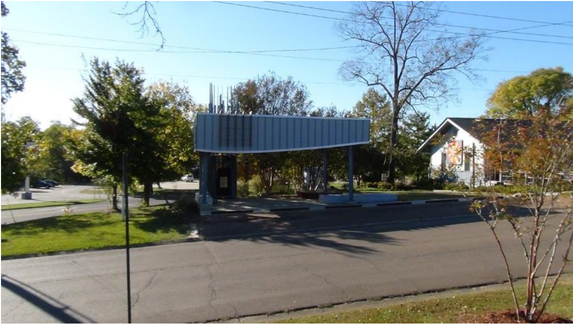
Figure 3.6 View of OCHM from vantage point two, approximately 34 m east of roof
