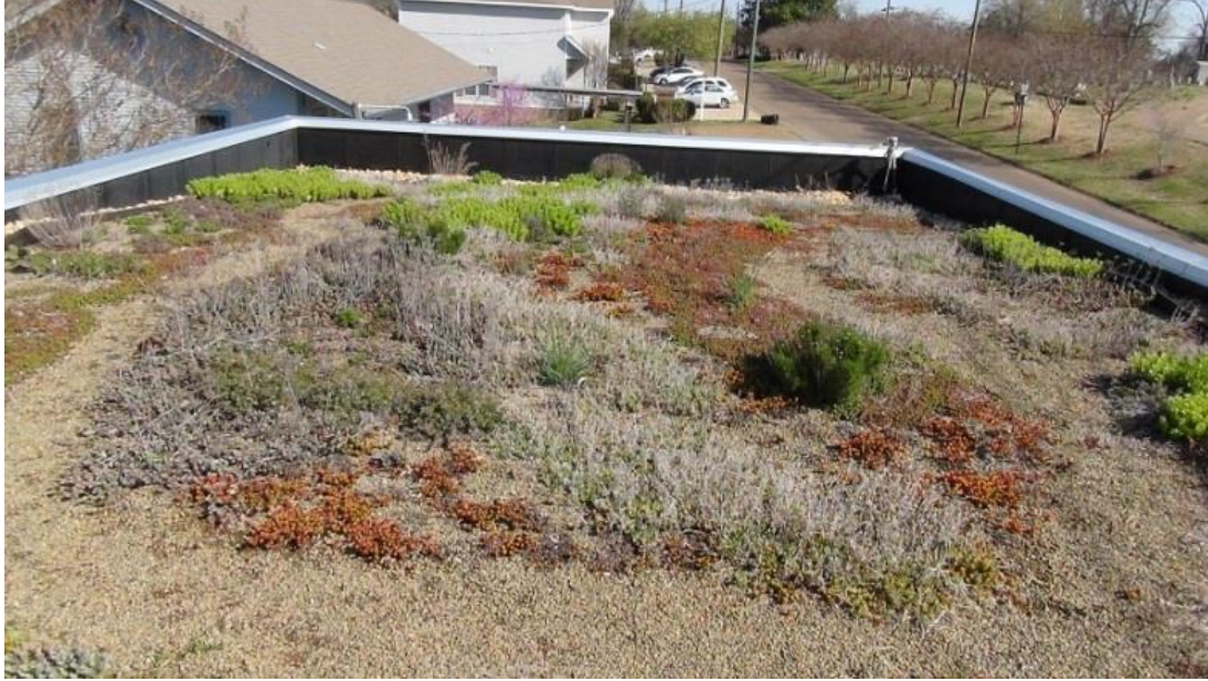
Figure 4.33 View facing north on OCHM green roof, March 2014
