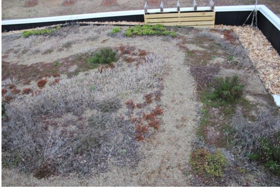
Figure 4.31 View facing east on OCHM green roof, February 2014
