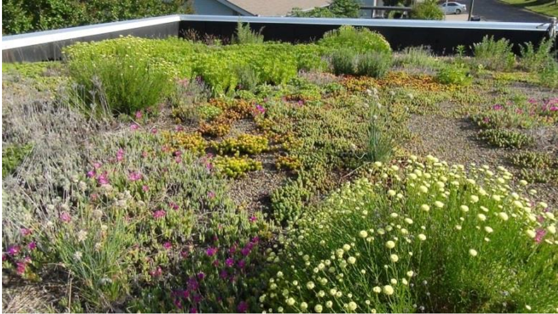
Figure 4.37 View facing north on OCHM green roof, May 2014
