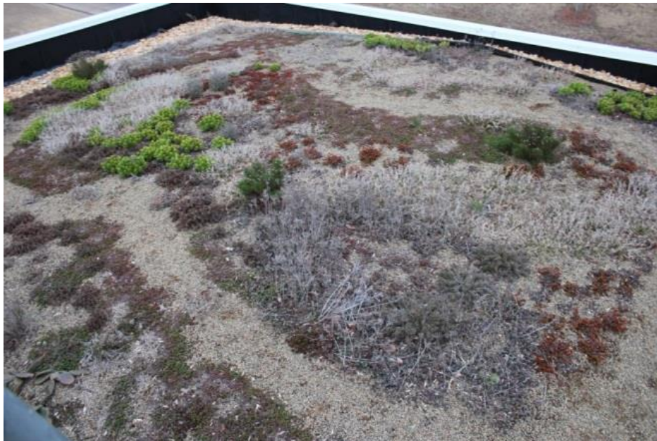
Figure 4.30 View facing northeast on OCHM green roof, February 2014
