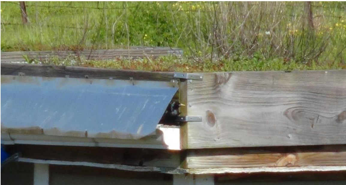
Figure 4.49 April 19, 2014: EUST investigates stormwater infrastructure on a Sedum roof
