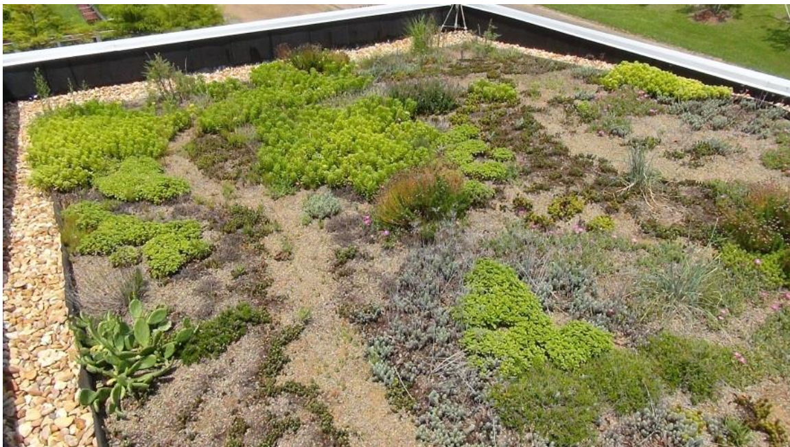
Figure 4.38 View facing northeast on OCHM green roof, July 2014
